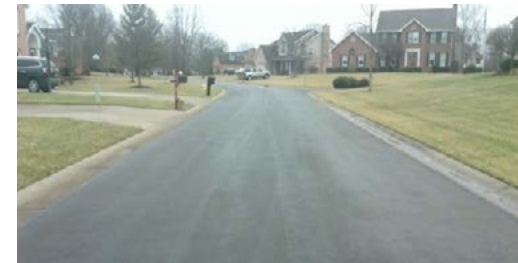
Thin overlay application on Clemray Drive
